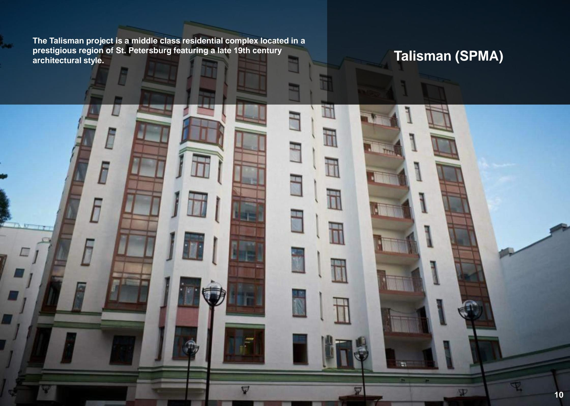
**Description:** Four 17- to 24-storey buildings using poured concrete technology with brick elements and ventilated facades.
