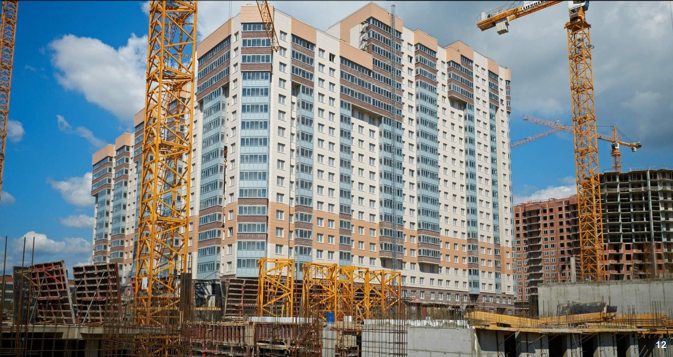
**Description:** Thirteen buildings up to 25 floors using poured concrete technology with brick elements and ventilated facades.
