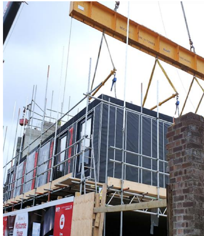
FINISHED MODULE INSTALLATION
