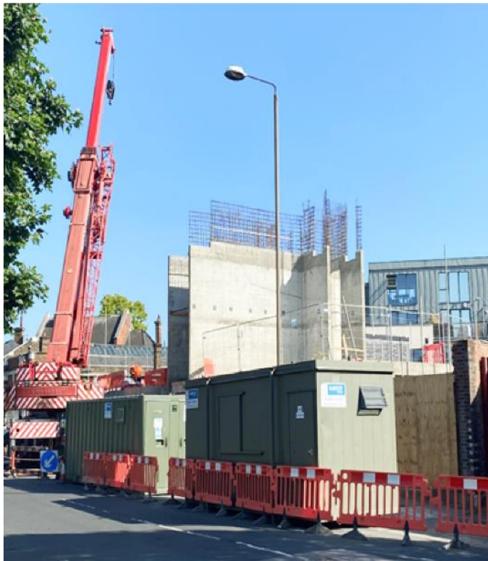
CAST-IN-PLACE CORE
