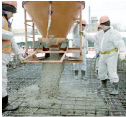
Poured-concrete construction typically involves the walls and slabs being constructed together by pouring fluid cement concrete into a formwork system, while using metallic reinforcement bars for strengthening and stabilisation purposes. Openings for doors and windows and electrical and plumbing elements are also in place before the concrete is poured.
