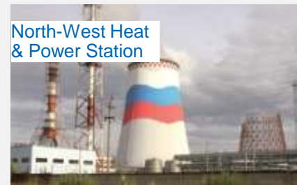
North-West Heat & Power Station Foundation construction for a cooling tower and main building
