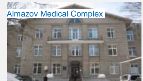
Almazov Medical Complex Renovation of the existing building and building up two additional floors
