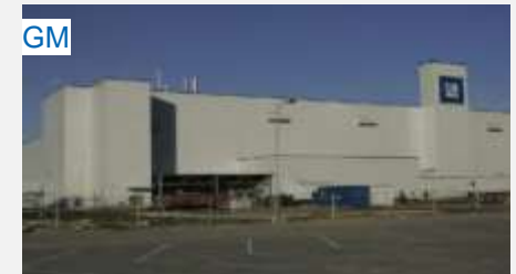
GM Poling & road infrastructure construction
