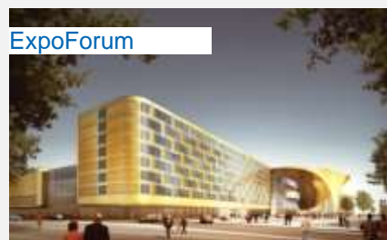
ExpoForum Full construction cycle
