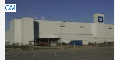
GM Poling & road infrastructure construction
