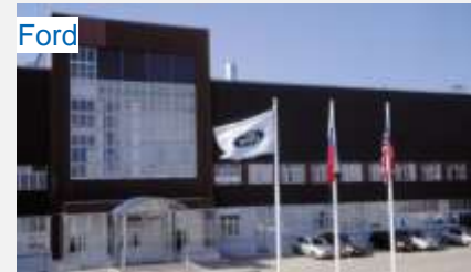
Ford Design & construction (increase of production capacities)
