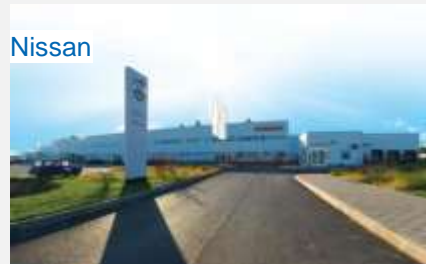
Nissan Infrastructure & site for the finished goods
