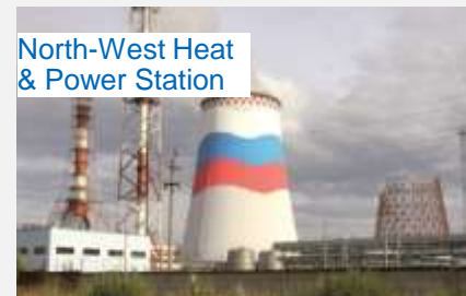
North-West Heat & Power Station Foundation construction for a cooling tower and main building
